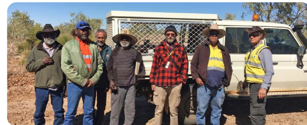
Above: Traditional Owners on site during construction of the NGP.
